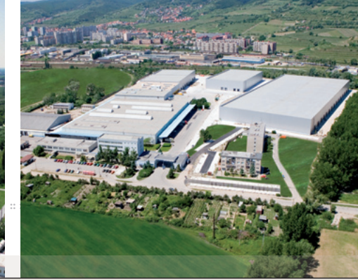
Logistics Center Bratislava – Rača
